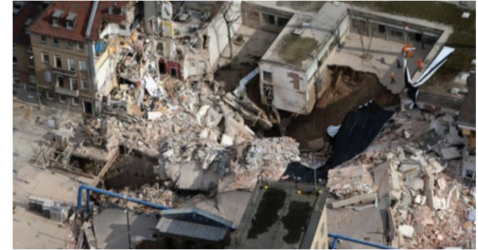
Collapse of multiple buildings resulting from excavation collapse, due to metro construction, Cologne, Germany. Source: National Research Council, 2013.
