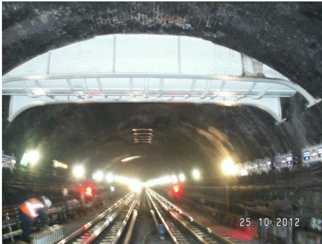
River passing through tunnel crown of a sub-surface tunnel.
