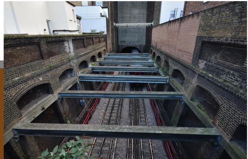
Typical cutting with building over cutting retaining wall, and building offset from top of retaining wall
