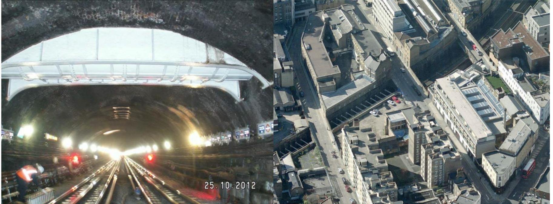
**Source:** London Underground, 2012. PC100, carrying the King's Scholars Pond Sewer, through the roof of tunnel TL53, west of Baker Street. [photograph] London Underground survey.
