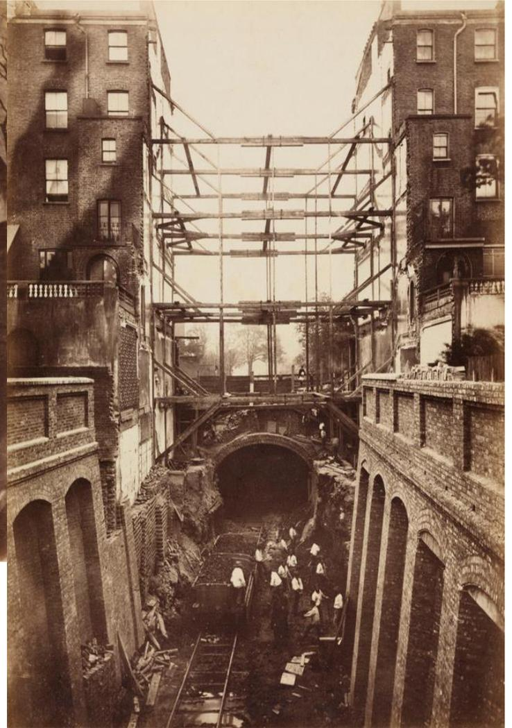
Photographs showing the construction of the Circle line between Bayswater and Notting Hill, to the rear of Leinster Gardens
