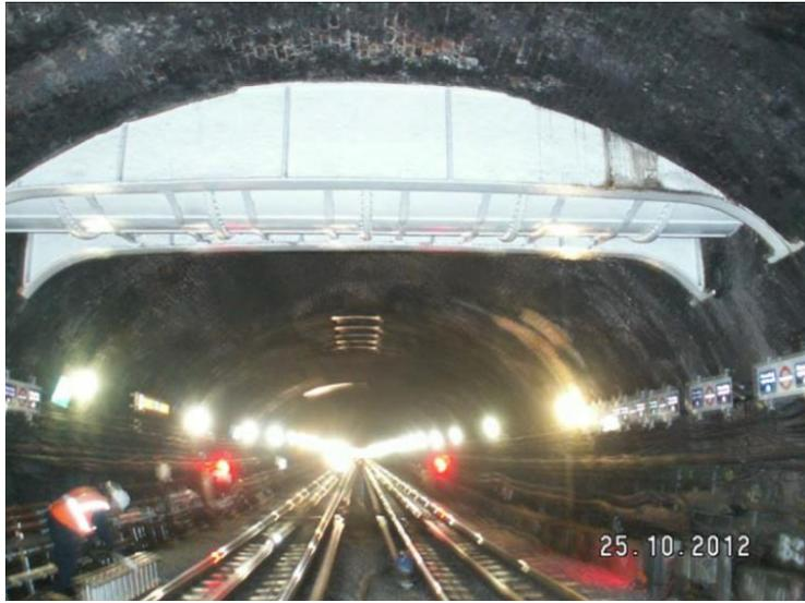
A river passing through the crown of a sub-surface tunnel
