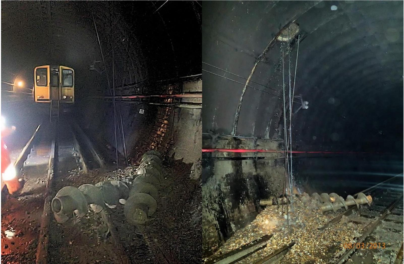
**Penetration of tunnel lining and auger sections and debris on the track**
