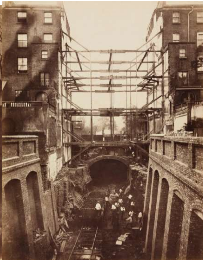
Photograph showing the effects of UUMI construction, Porchester Terrace, London. Source: The Sun, undated.
