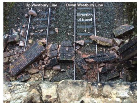
Fallen bridge parapet at Froxfield, 2015. Source: RAIB, 2016
