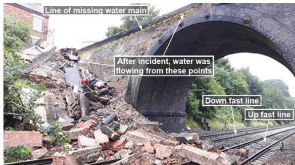
Partial bridge collapse, Barrow Upon Soar. Source: RAIB, 2017a.
