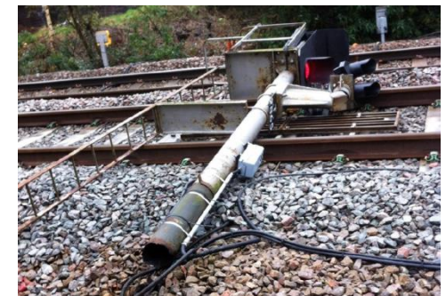
Collapsed signal post at Newbury. Source: RAIB, 2015.
