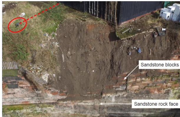
Retaining wall collapse, Liverpool 2016. Source: RAIB, 2017b.
