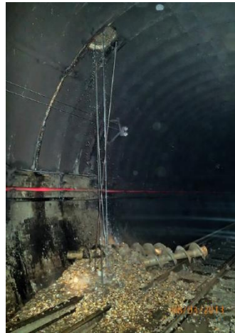
Tube tunnel penetration, London, 2013. Source: RAIB, 2014.
