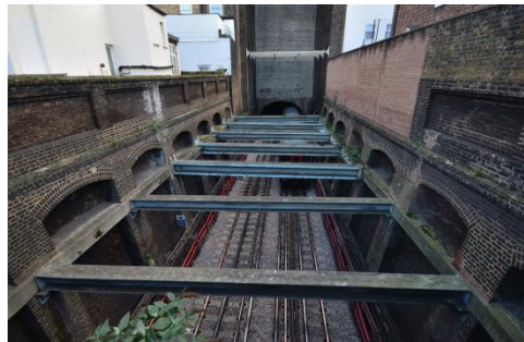
Buildings above retaining walls; Props supporting the retaining walls
